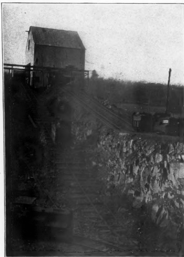
Inclines to the Primary Crusher
